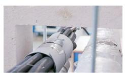
Apply two layers of bandage and fix them with an overhang of 75 mm.
