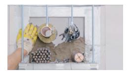
Mix the coating material, pre-wet the reveal, insert cables into the sealing area with the mortar, and smooth the surface.
