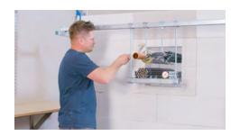
Clean the reveal of the structural opening and installations and mask them with adhesive tape.
