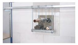
Remove the adhesive tape, clean the work area, and label the seal.
